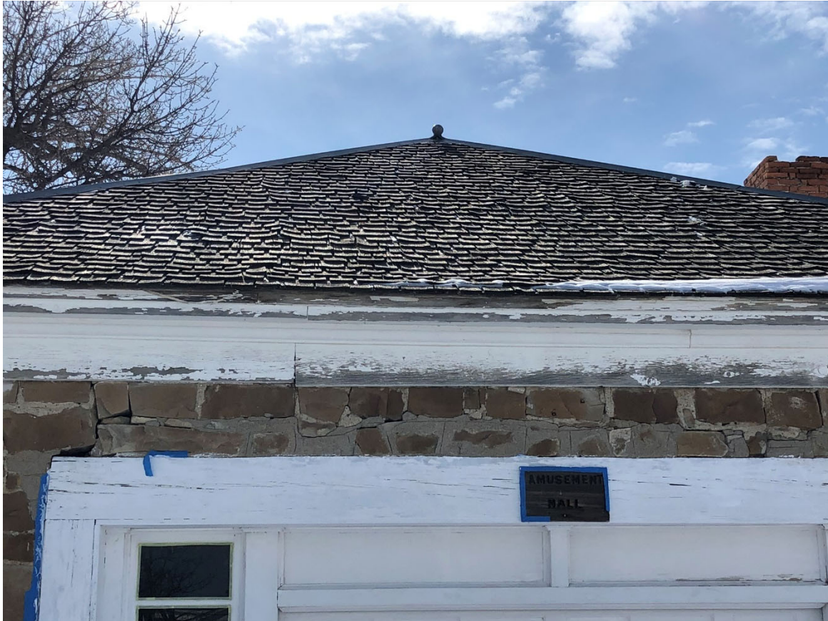
A. EXISTING WOOD SHAKE ROOF & FASCIA DAMAGE, WEST ELEVATION-LOOKING EAST
