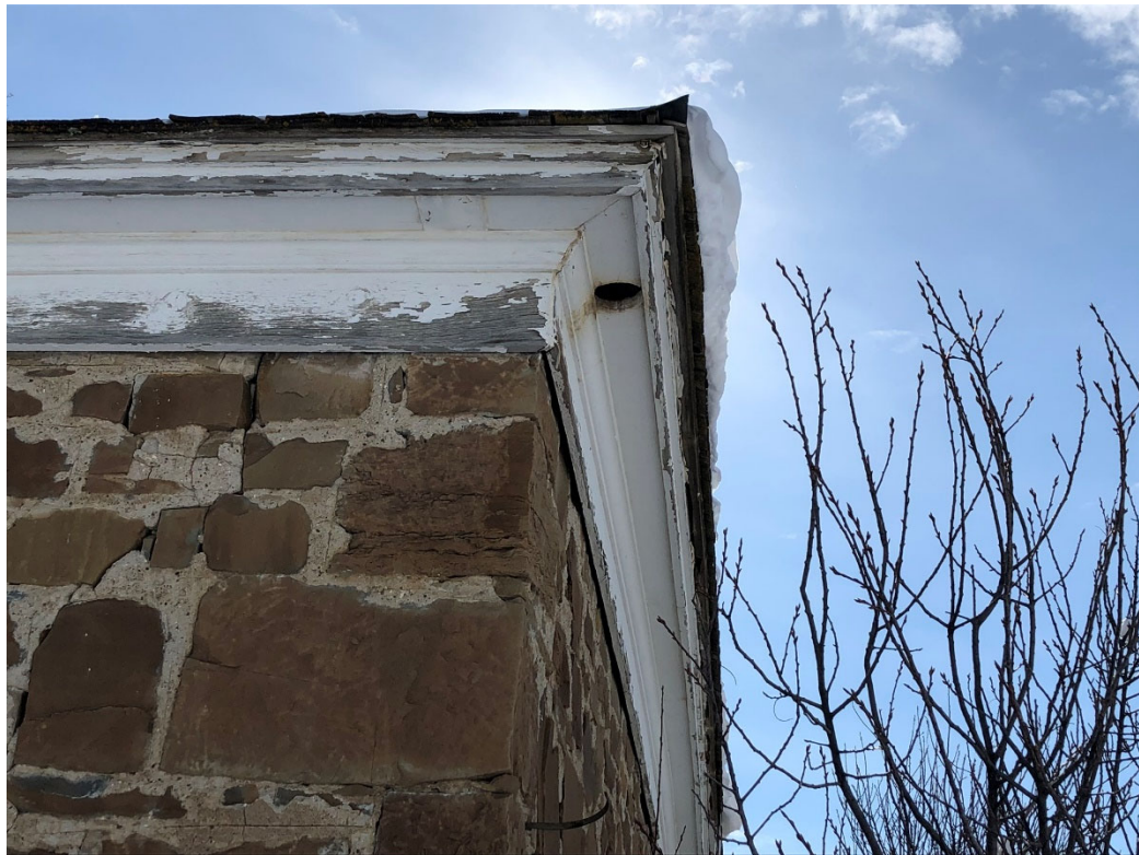
F. FASCIA REPLACEMENT AREA, WEST ELEVATION-LOOKING EAST
