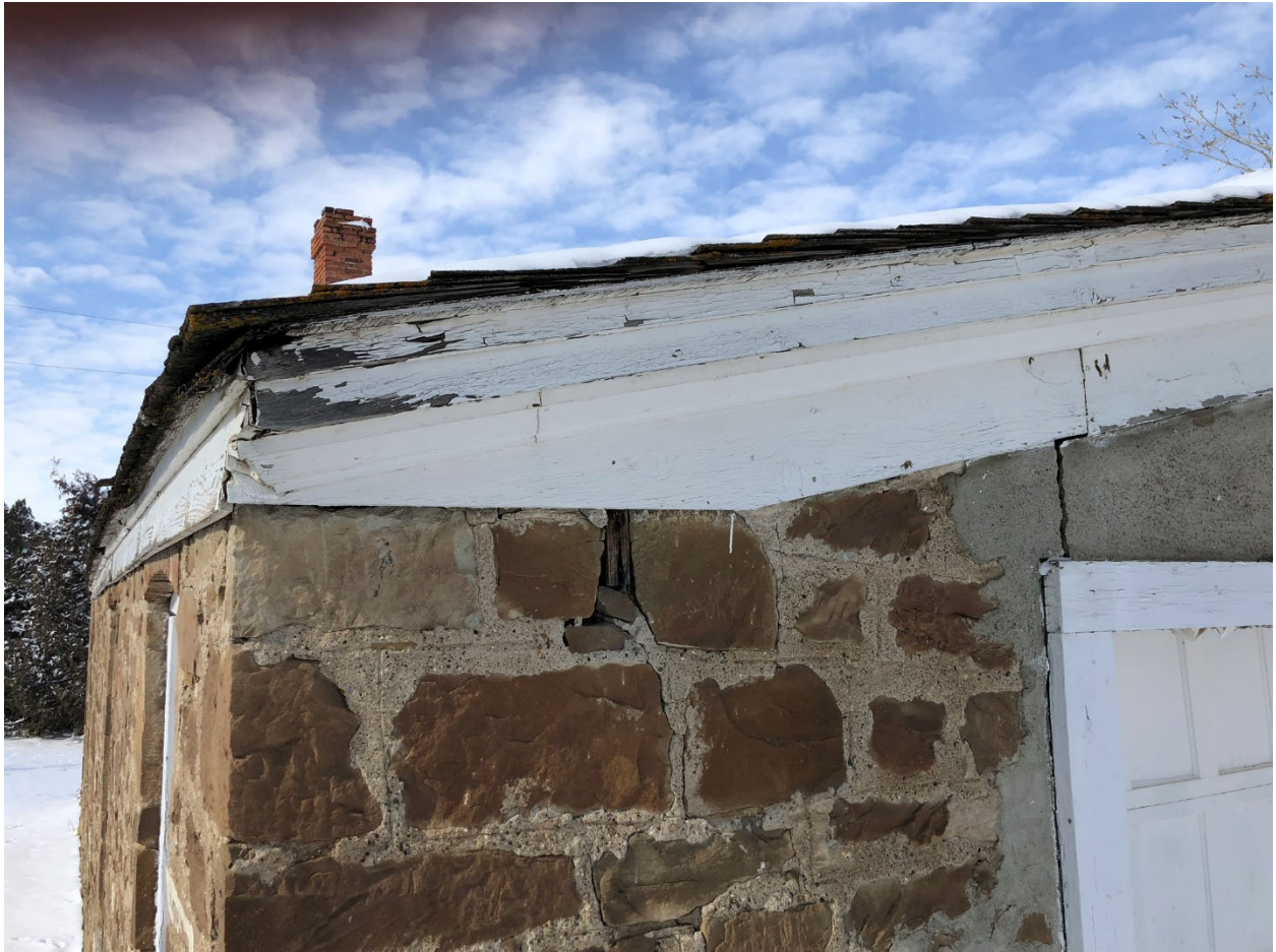
G. FASCIA REPLACEMENT AREA, EAST ELEVATION-LOOKING WEST
