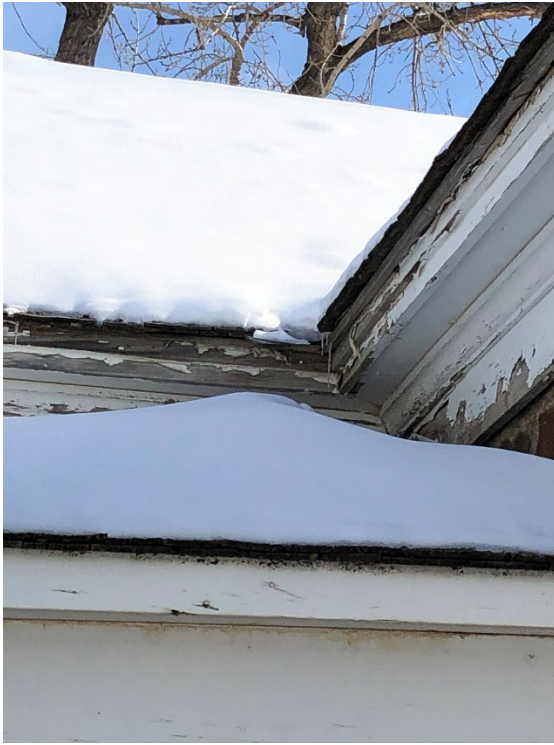
E. FASCIA REPLACEMENT AREA ABOVE PATIO ROOF/DOOR, SOUTH ELEV.-LOOKING NORTH
