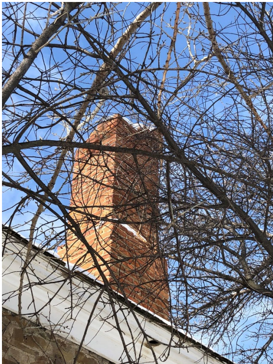
D. NORTH CHIMNEY
